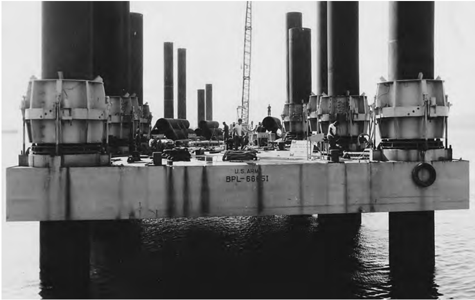
DeLong pier at Cam Ranh Bay nearing completion, December 1965
